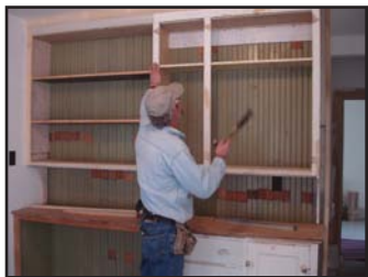
Denny Weis installed the antique kitchen cupboard.
