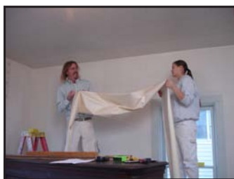
Jay Ryan and Corrine Ryan Seymour hanging the ceiling wallpaper in the front parlor.
