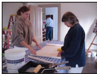
Corrine Ryan Seymour and Marilyn Ryan cut and prepare the wallpaper for application.
