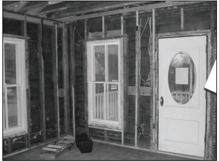
View of the dining room before new insulation.
