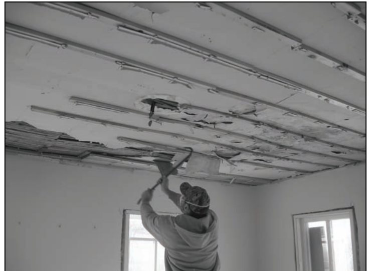
The ceiling was carefully removed in layers in each room.
