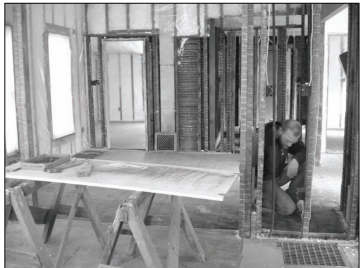
Joel Berglin removes the flooring down to the original floor. January 2007
