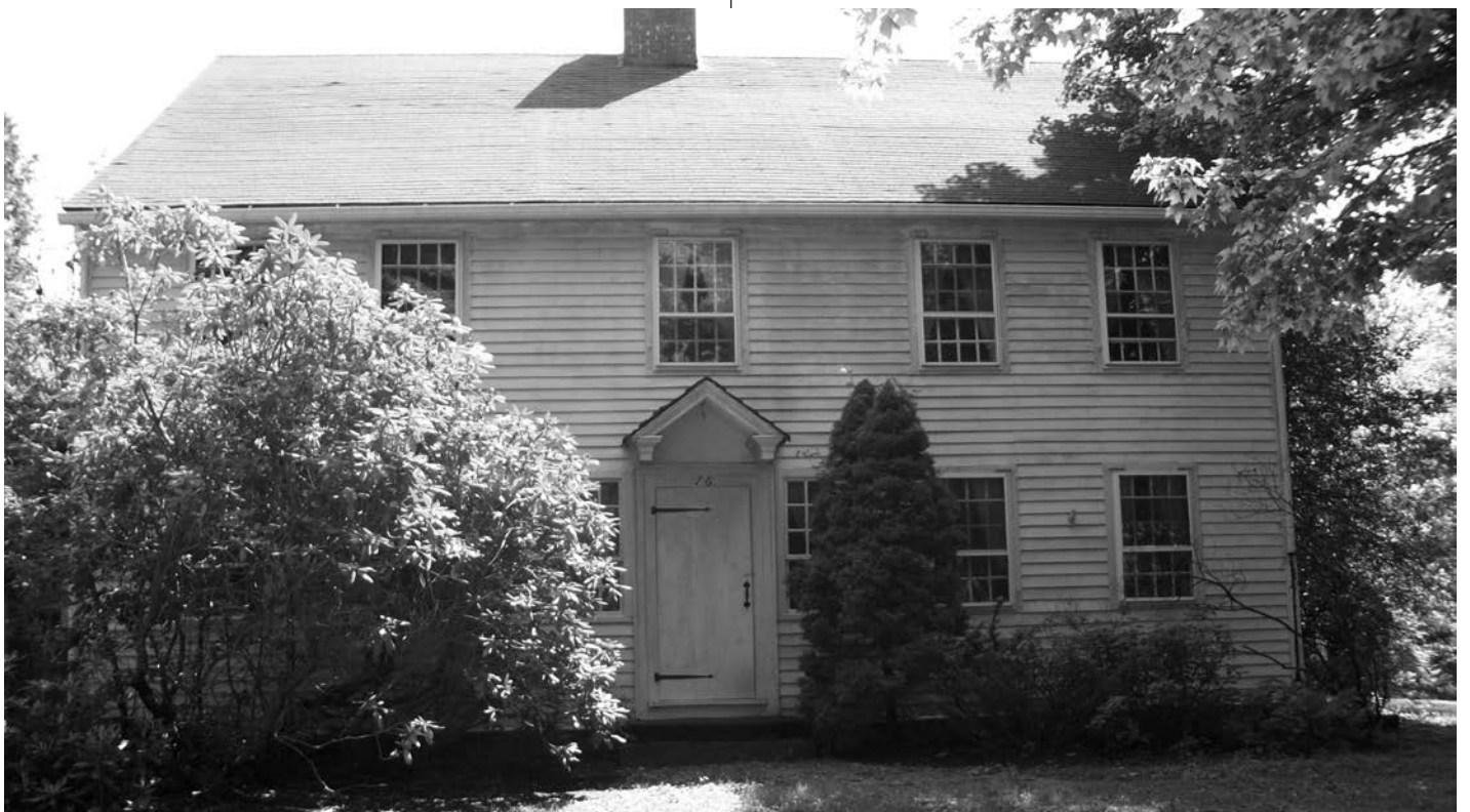
Home of author and illustrator Lois Lenski Covey in Harwinton, Connecticut. In the early 1930s, Lois and her husband Arthur moved into this early American house on Harmony Hill Road. They called this old abandoned farmhouse and neglected outbuildings “Greenacres”. (Photo courtesy of Kathleen Baxter, 2013)
