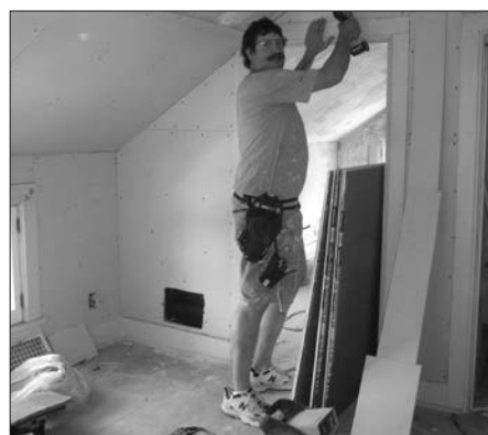
Candy and Doug Laven installing new sheet rock.
