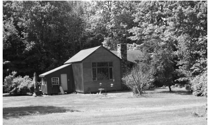
“In 1935 Lois even had the outbuilding south of the house that had once served as the Balch coffin shop renovated to serve as her studio.” Quote from Lois Lenski Storycatcher by Bobbie Malone This studio is where Lois created the illustrations for the first four Betsy-Tacy books. (Photo courtesy of Kathleen Baxter, 2013)
